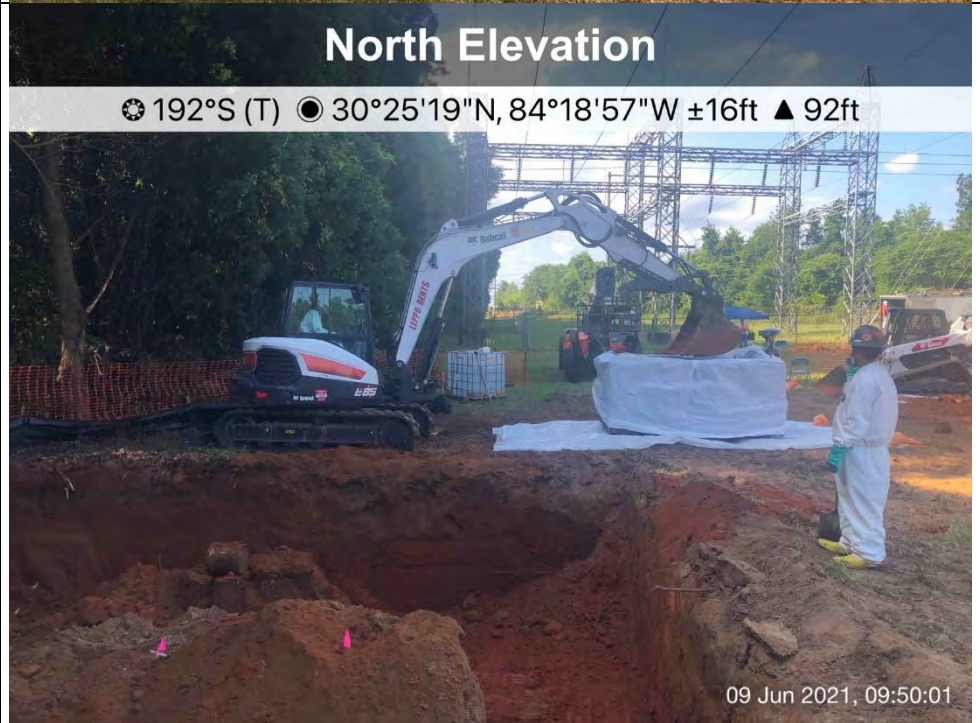
Photograph 2 LLRW excavation into waste bag.
